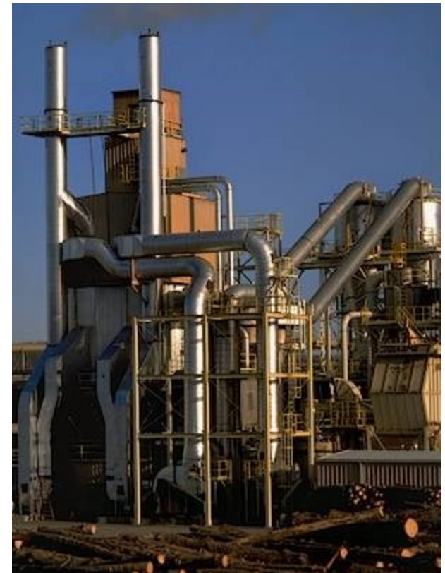
Scrubber at work
